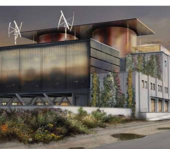
on all roofs, vertical wind turbines, heat pumps, ambient heat from an adjoining port basin, the ground and the air, together with waste heat from surrounding companies, is to be stored in the energy control centre. The intention is for the whole area including the new business site Piek 17 to become self-sufficient to a significant extent in terms of power, heat and possibly refrigeration.
