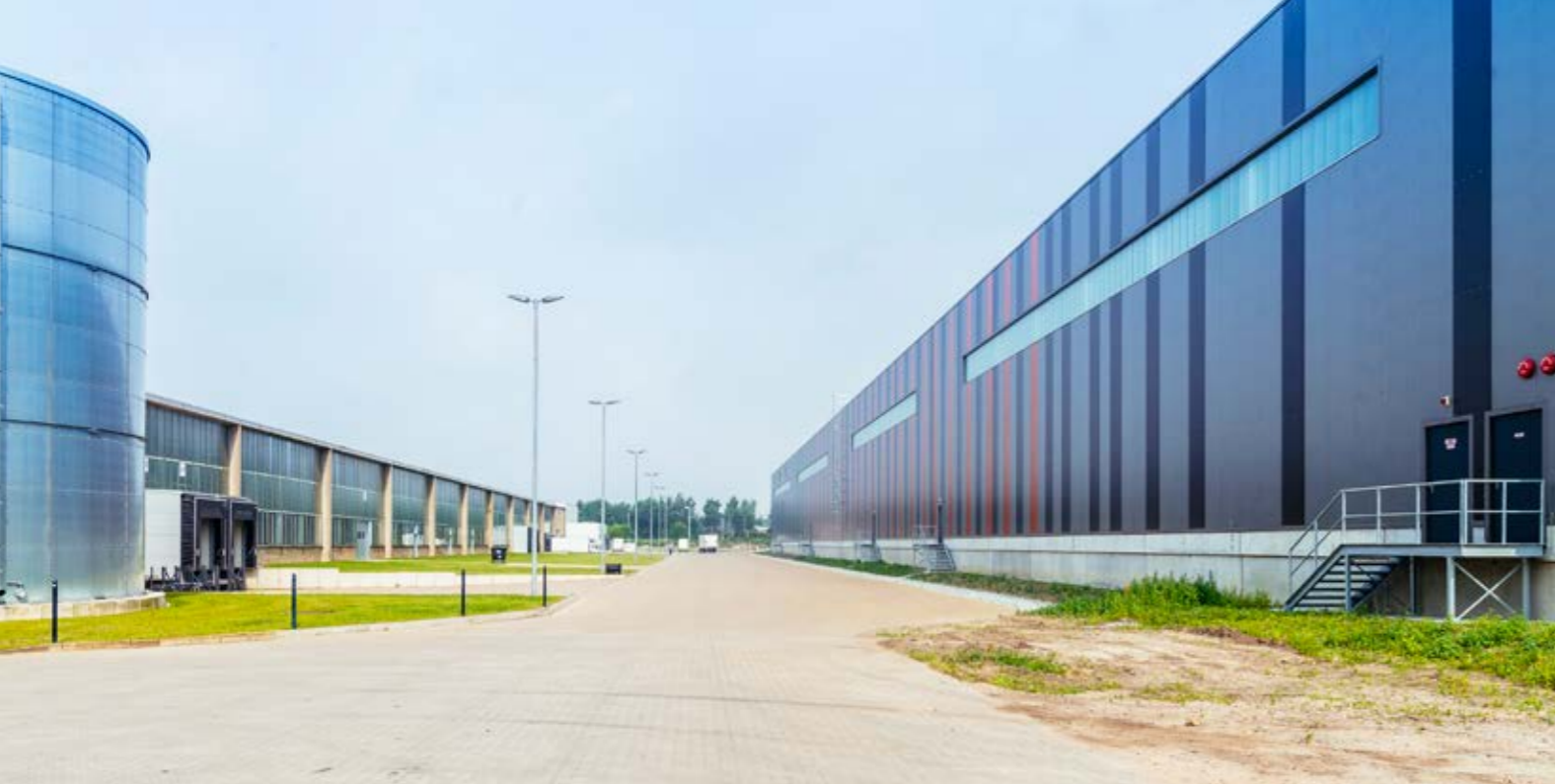
Lloyd Industriepark, Airport-Stadt-Nord
